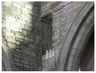
joists are certainly plenty big enough. There is an opening in the east corner of the south wall of the nave which could have provided access to the gallery, itself being reached by stone or wooden steps — now gone. If the current pointed arch was inserted later, the large opening would have had to be filled in to provide strength, and the small door would have provided access.
