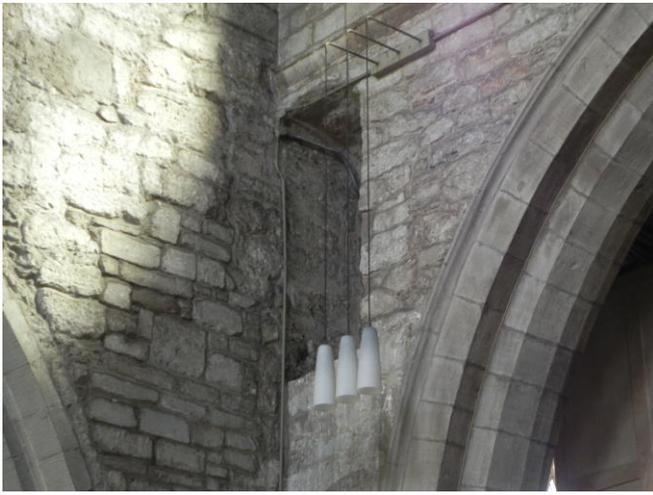
joists are certainly plenty big enough. There is an opening in the east corner of the south wall of the nave which could have provided access to the gallery, itself being reached by stone or wooden steps – now gone. If the current pointed arch was inserted later, the large opening would have had to be filled in to provide strength, and the small door would have provided access.
